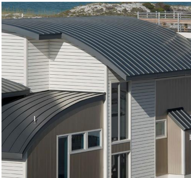
6. Standing seams metal vaulted roof (DARK GREY)
